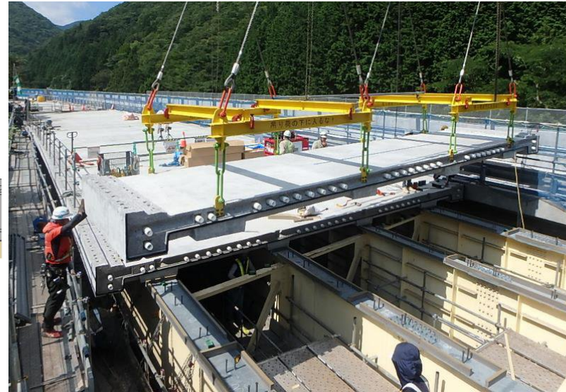
Installation of panel
