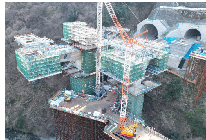
Nakatsugawa Bridge (Under construction)
