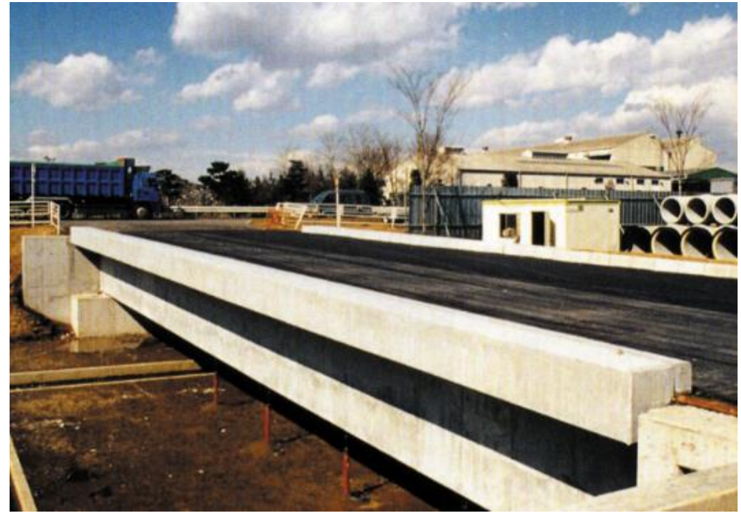
Post-tension beam (Non-metallic tendon)
