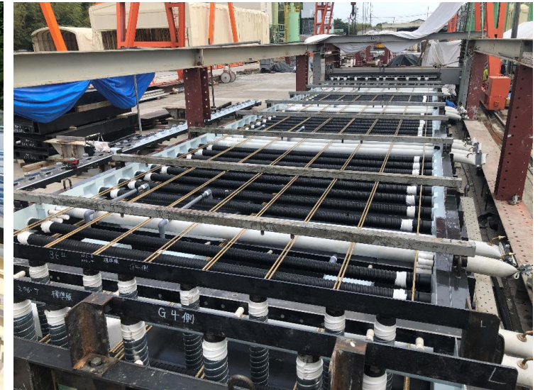
Prefabrication of Dura-slab pretensioned aramid FRP
