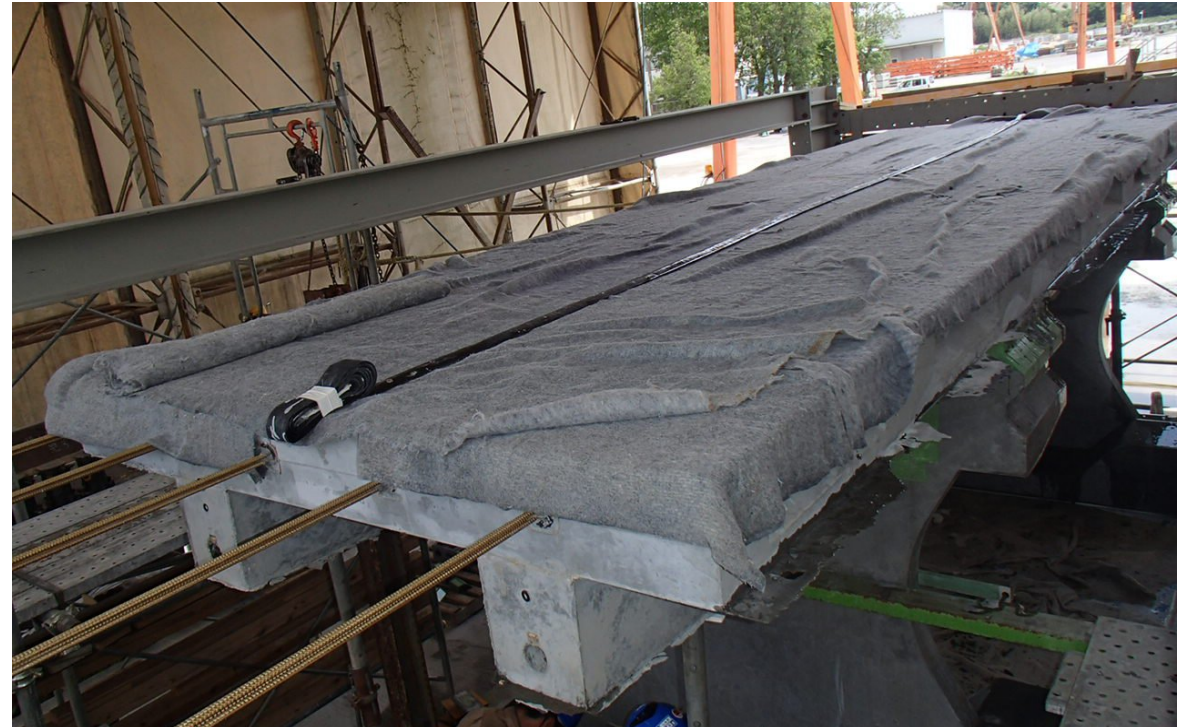
Fabrication of upper deck
