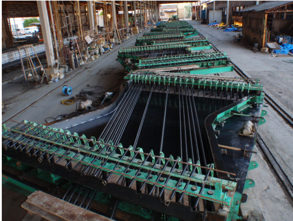
Pretension steel strands
