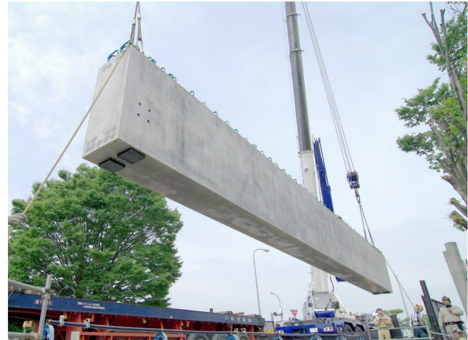
130 MPa concrete without Portland cement & aramid FRP tendons
