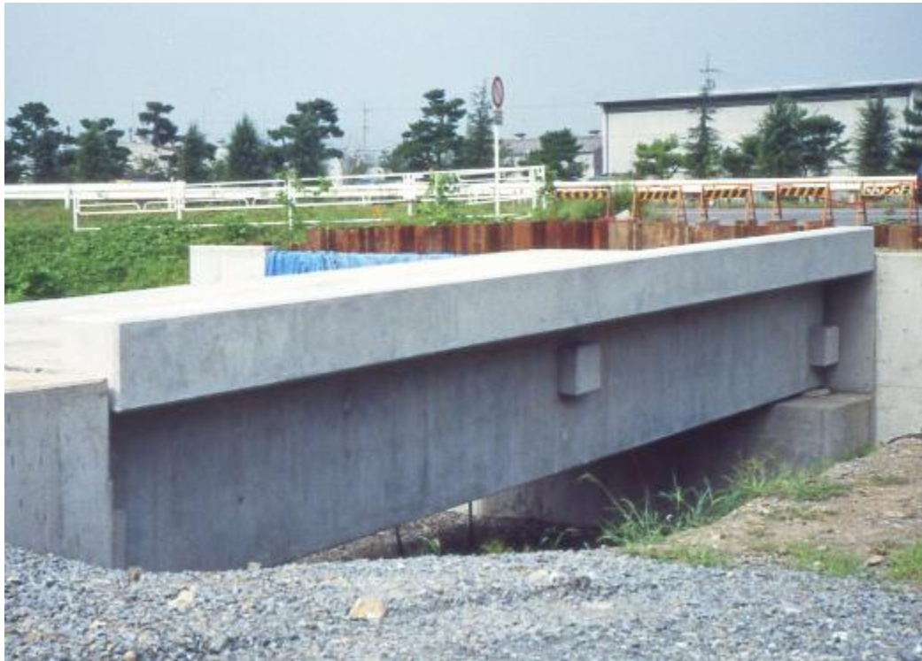
Pre-tension beams (Non-metallic bridge)
