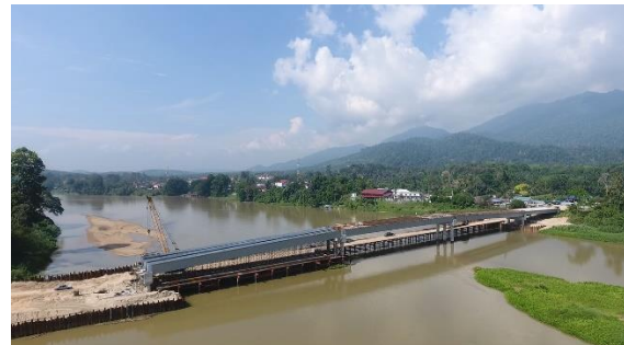
Fig. 8. Manong Bridge, Malaysia
