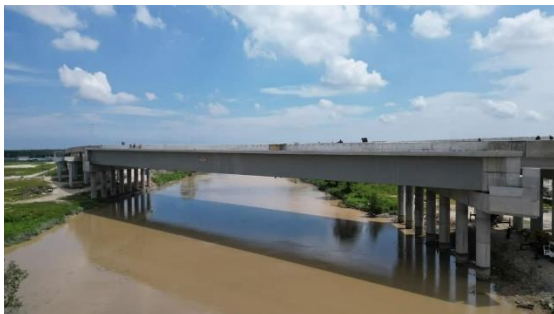
Fig. 5. Langat River Bridge (105 metre span)
