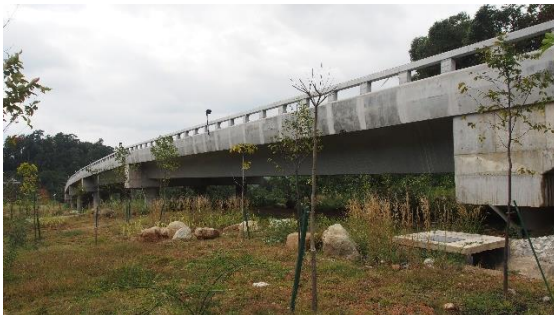
Fig. 7. Gerik-Kota Bahru Viaduct, Malaysia
