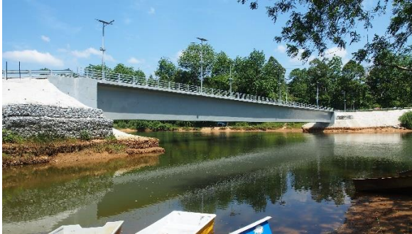
Fig. 1. Batu 6 Segmental Box Girder Bridge
